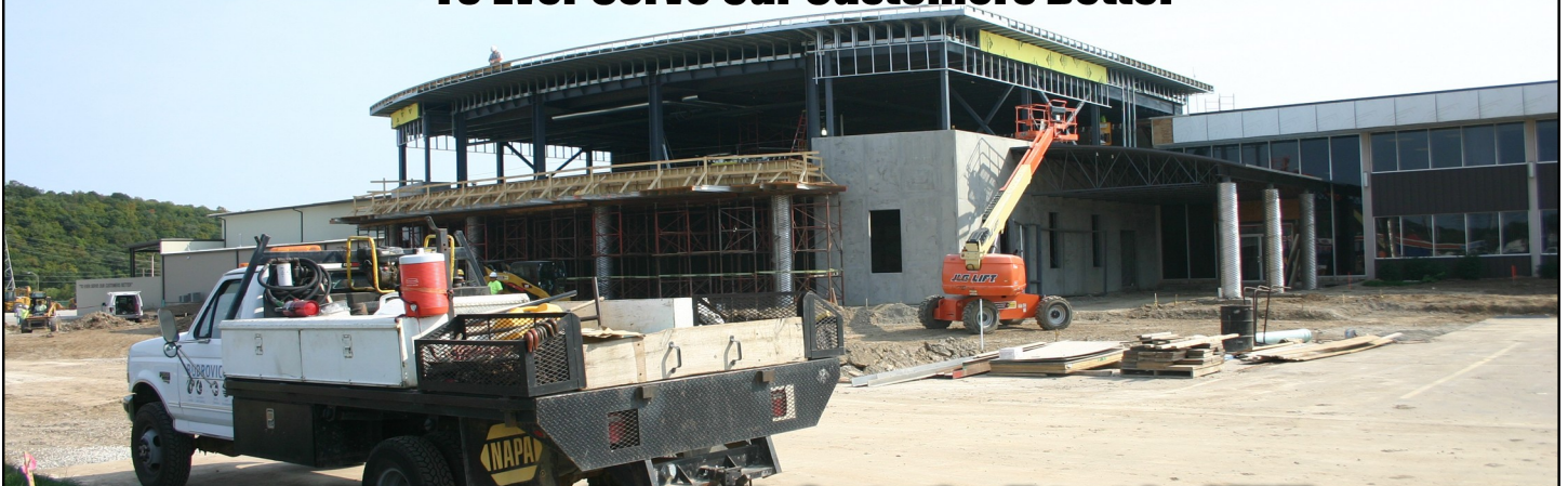
Building Expansion - Phase 2 Under Construction - Picture taken 9/25/12
